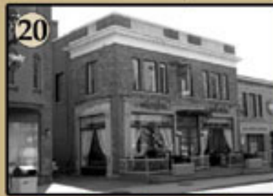
20 La Southern Canada Power 116, rue Principale
